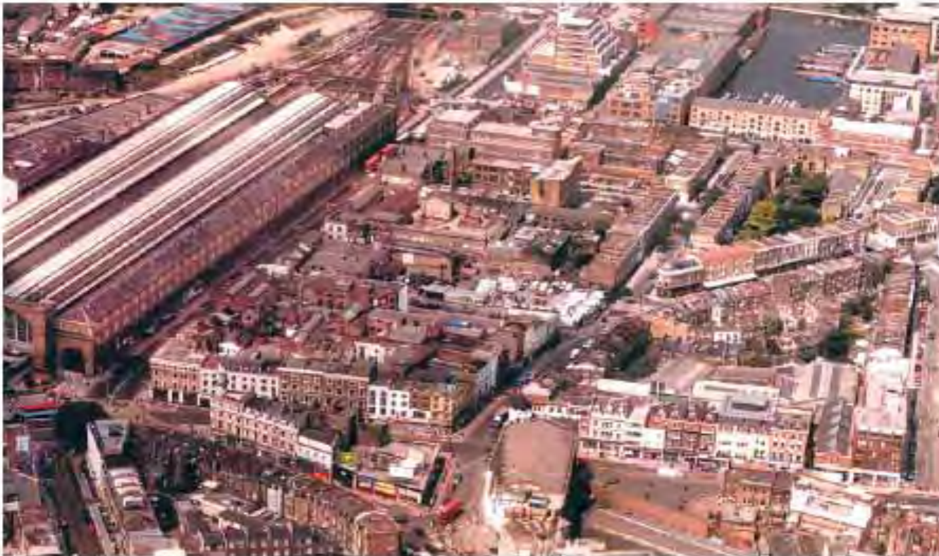
Figure 15, view of the east side of King's Cross before re-development (source data: Brochure one master planning, P&O – RHWL Architects, August 2001)
